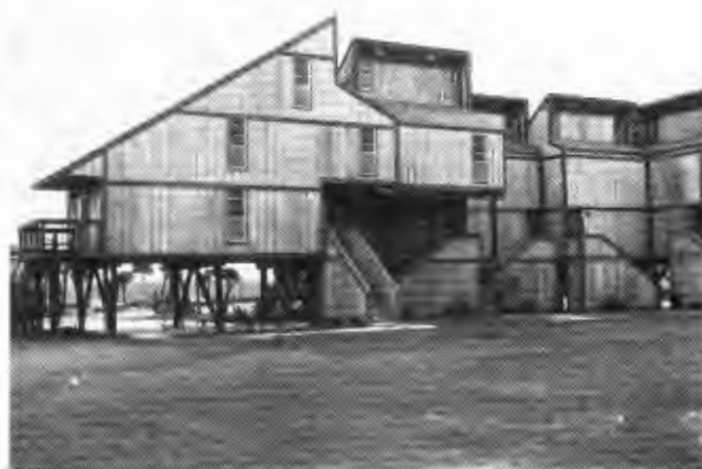
Figure 4.4. Elevation by Posts
