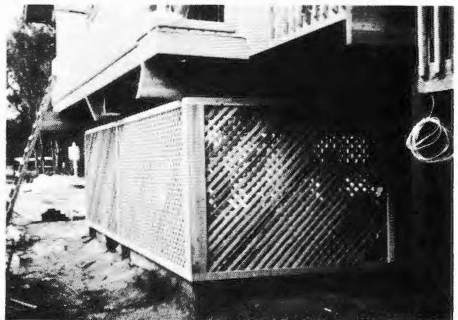
Figure 4.54. Breakaway Walls
