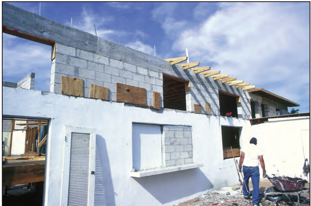
Figure 67 The extended first-story walls.
