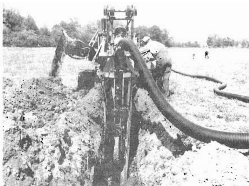
Figure F-1. Installing plastic tubing for a subsurface drain.
