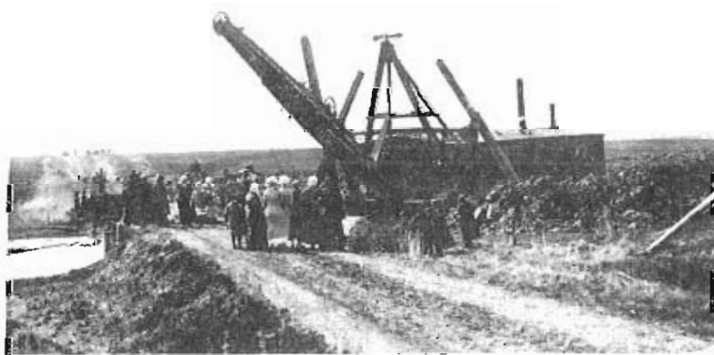
Figure 2. Floating dredge excavating a drainage ditch in 1904.
