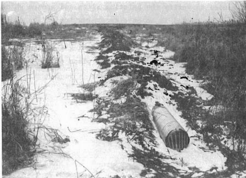
Figure H-1. A recently installed subsurface drainage outlet.
