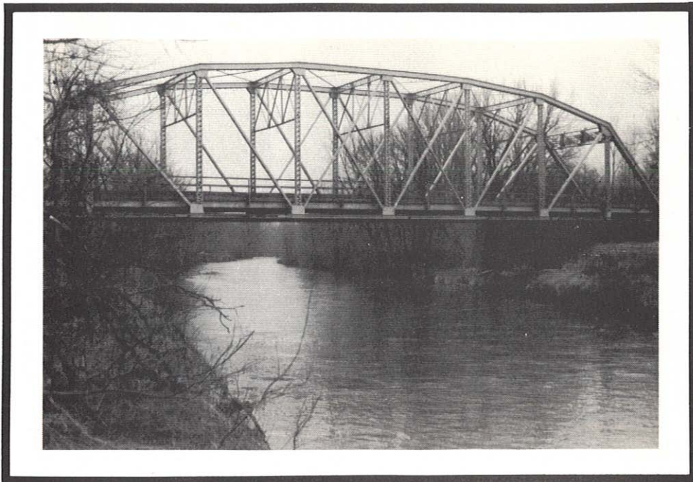
Figure 5. Skunk River - Iowa Highway No. 221, looking upstream, Mile 16.75.
