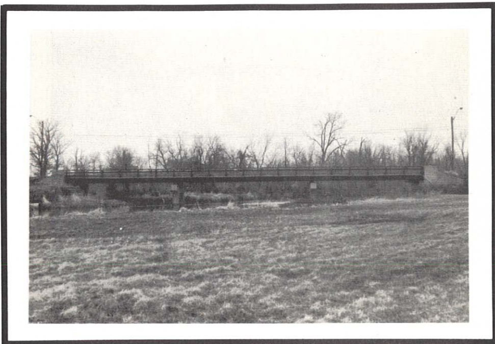
Figure 6. Skunk River - Broad Street, looking downstream, Mile 20.67.
