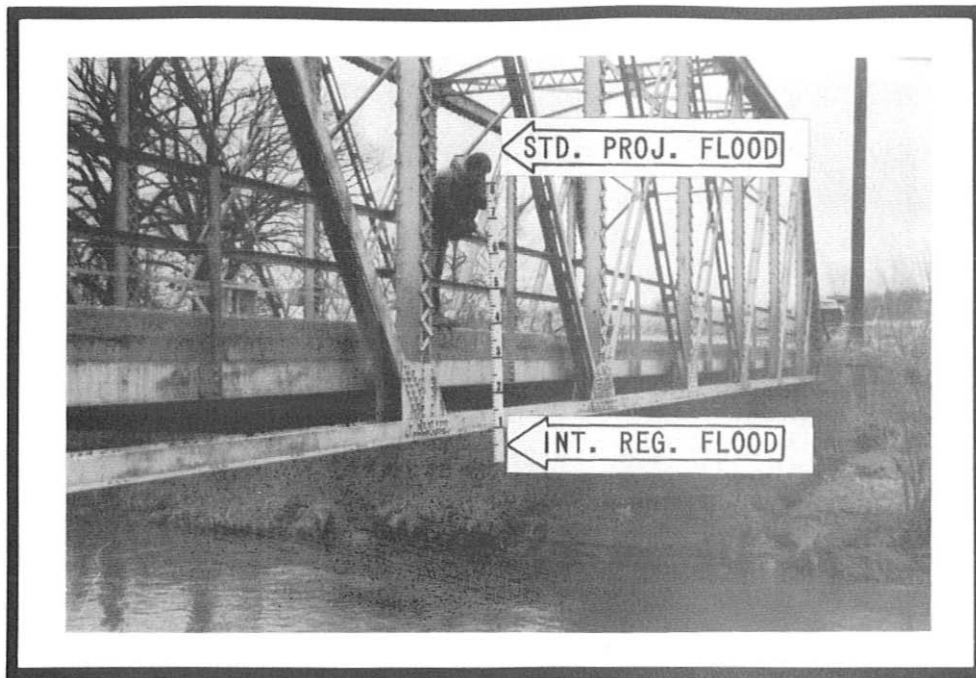
Figure 12. Skunk River - county road, northeast corner of Section 13, T84N-R24W, Mile 8.02, downstream side.
