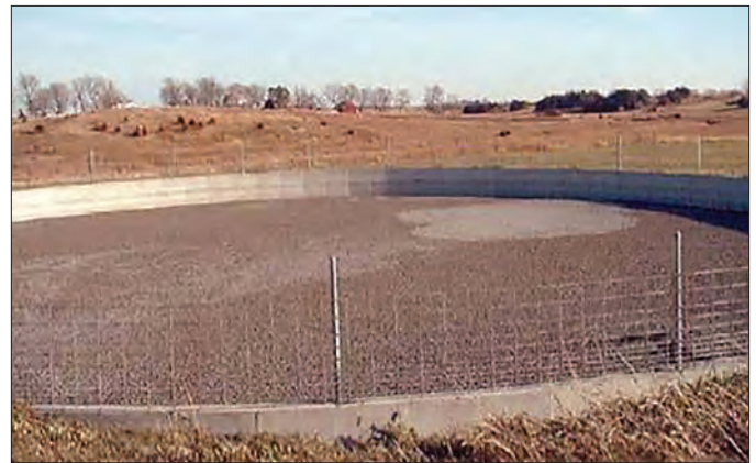
Figure 1. Lightweight expanded clay aggregate (LECA) permeable cover on an in-ground concrete swine manure storage tank. LECA covers are typically applied in a 2 to 4 inch layer.
